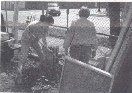
UI Architecture students volunteered to clean and organize the Salvage Warehouse. They also help salvage hundreds of pieces of tin ceiling. photo by D. Leasure
