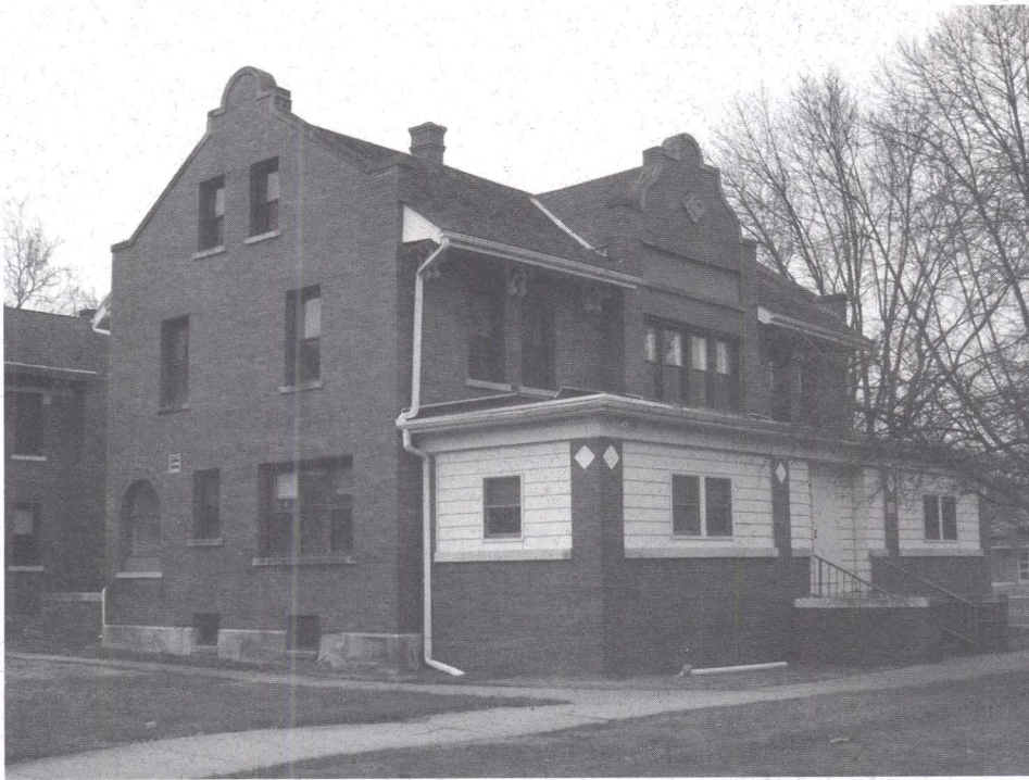
Jacobean Anglo-Dutch style gables distinguish the farm superintendent's house.
