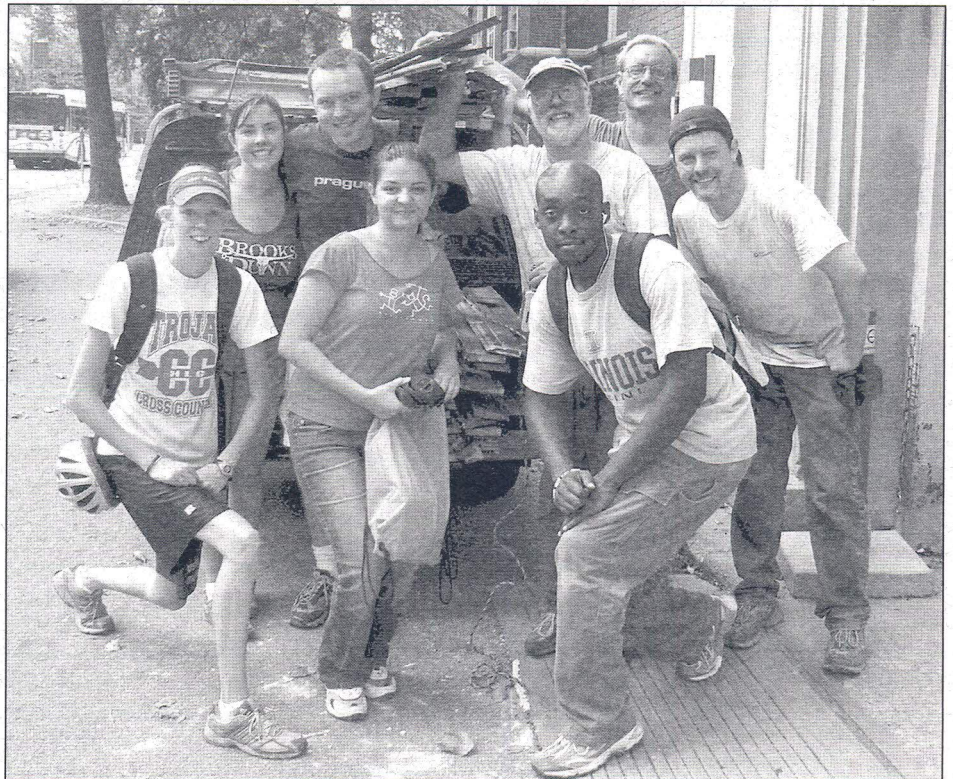
UI students from the Society of Architectural Historians spent a long day salvaging during the remodeling project in Noyes Lab. Most of the doors, trims, etc., are now part of the Blind Pig Pub in downtown Champaign.
