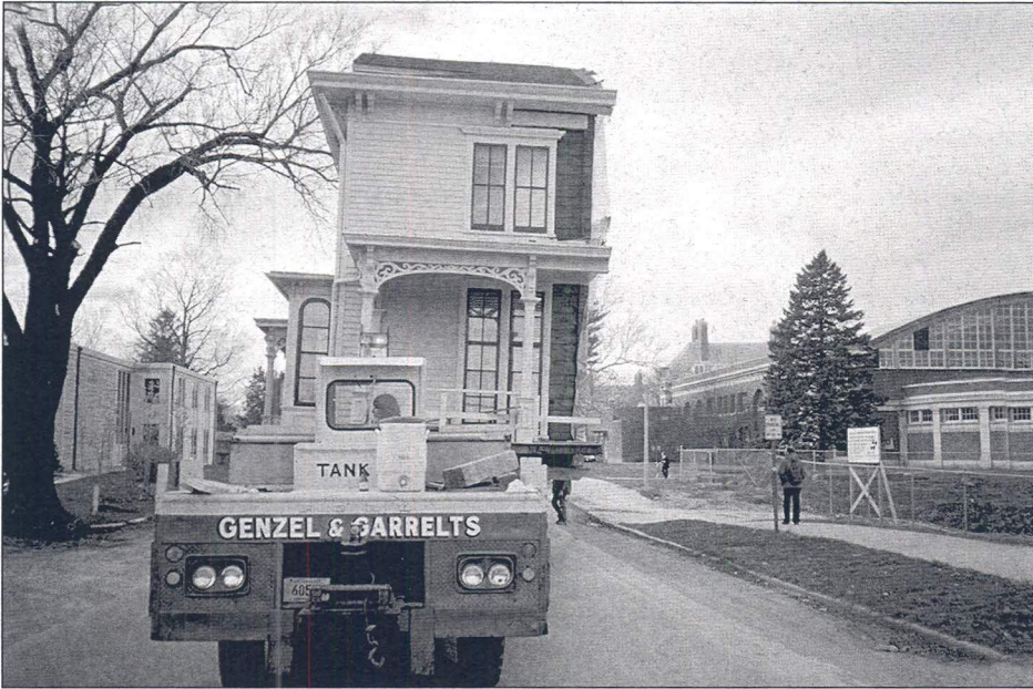
The Lorado Taft House was cut in half before moving it down Pennsylvania Avenue. The Stock Pavilion is in the background.
