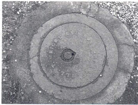
Cistern Lid from Wright foundry (In yard of Urbana house built in 1899)
