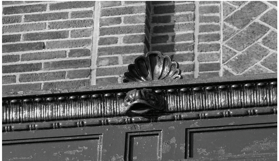
Detail of cast iron marquee on the South entry
