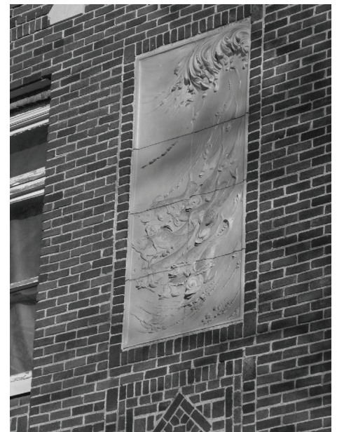
Ceramic plaque, west side of building
