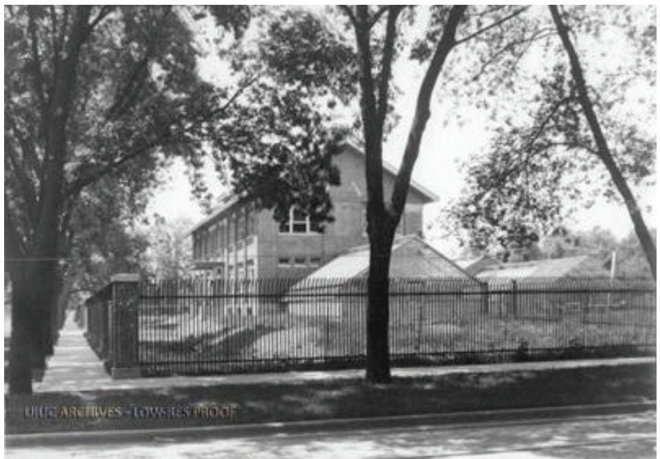
1926 view from the SouthEast
