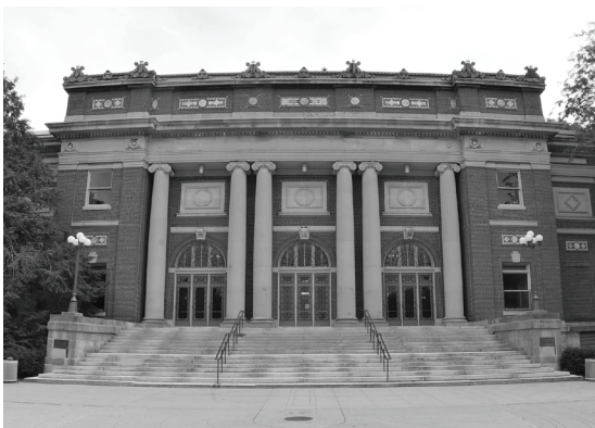
The steps before renovation (left), and today.
