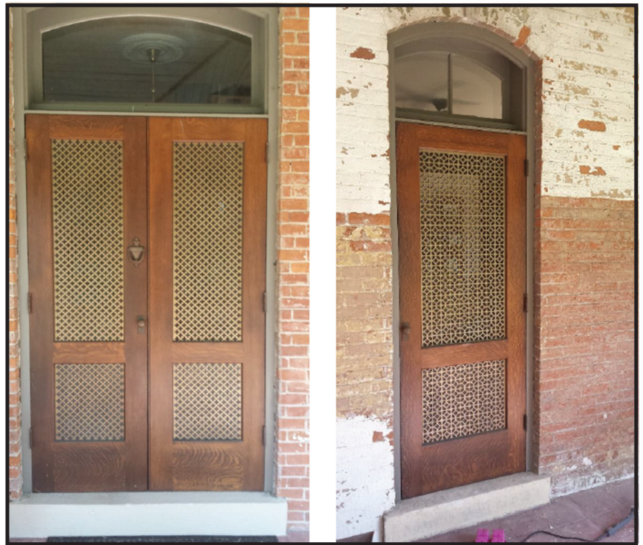
Henson House, Villa Grove, Illinois. Arts & Crafts Entrance doors produced by the Higgin Manufacturing Company of Newport, Kentucky.
