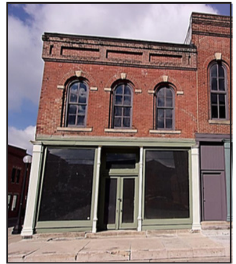
Former "Centennial Saloon" (1878-1879), 201 N. Market St
