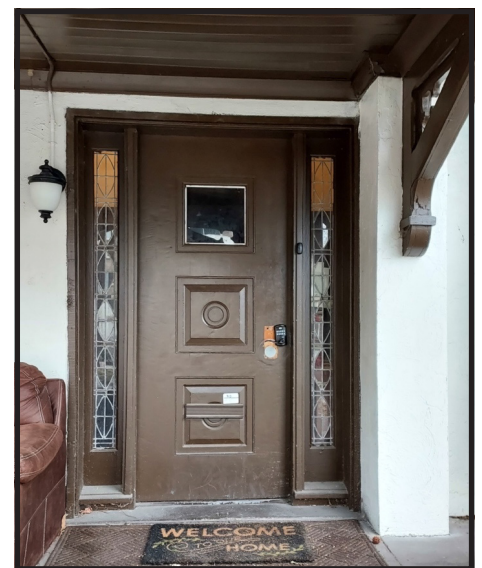
Entrance door, north elevation.
