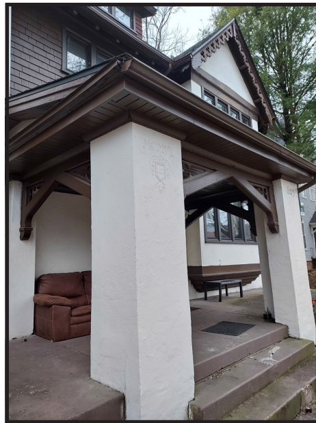
North elevation, porch detail.
