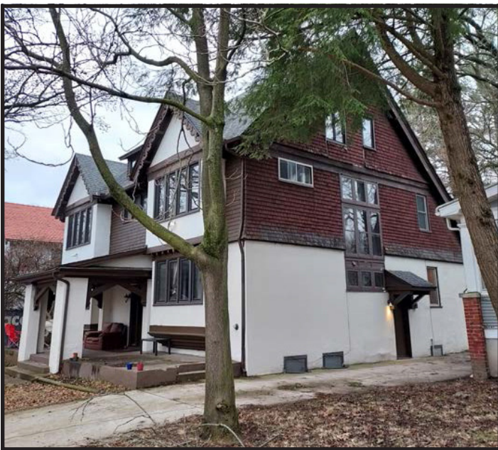
West and north elevations.
