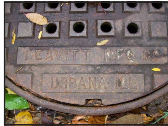
Manhole Cover in Champaign produced by the Leavitt Mfg. Co. of Urbana
