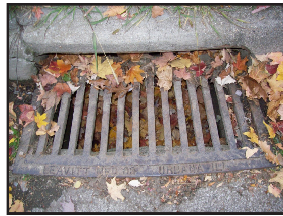
Storm Sewer Grate produced by the Leavitt Mfg. Co. of Urbana, Clark Park neighborhood, Champaign
