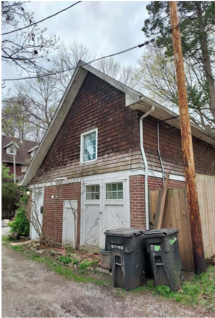
Carriage house/garage, east and north elevations.
