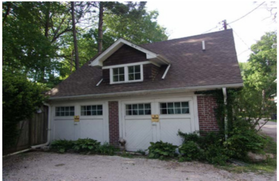
Carriage house/garage, south elevation.
