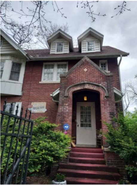
Parapeted east entry porch.
